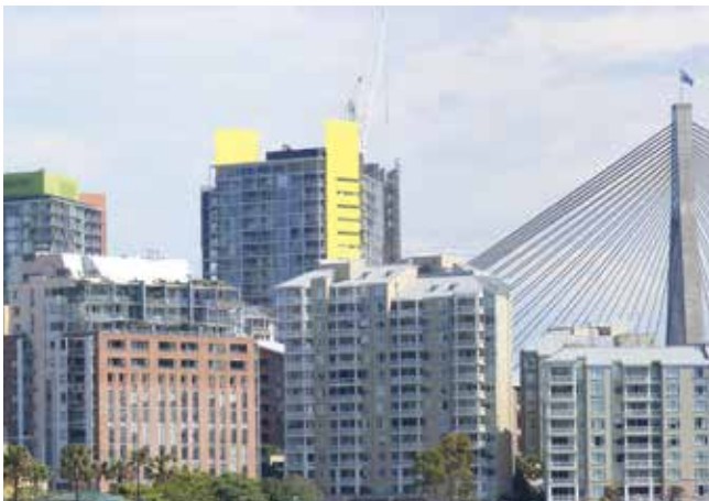
JACKSON LANDING, PYRMONT NSW
